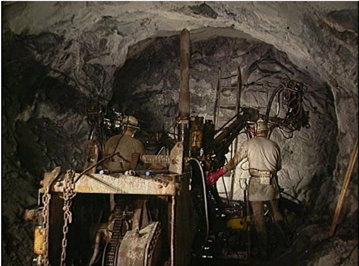
Figure 5-6: Photography of Drill and Blast driving in Haje [40]
