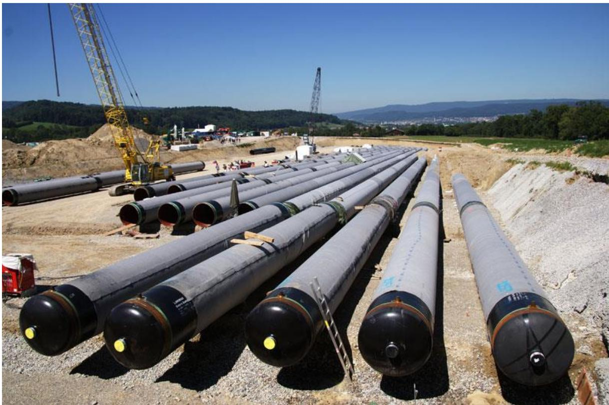
Figure 7-1: Photography of pipe storage construction workings for the Zürich Transport AG [40]
