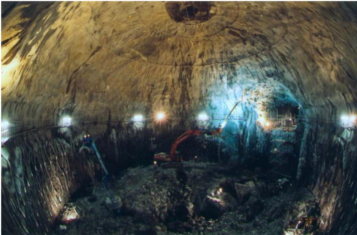
Figure 5-7: LRC Skallen, photography of partly excavated cavern [41]
